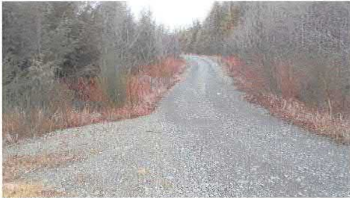
3) Access road near the Phase 1 and 2 Highlands Housing Site.
